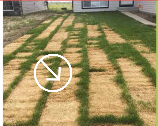
SOD THAT HAS NOT BEEN INSTALLED UPON DELIVERY
